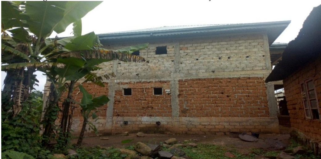
Figure 1: Showing a Blend between a Cement Block and Sundry in a G-Plus 1, around Foncha Street
